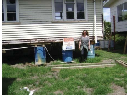
WASSTB CEO, Liz Andrews on site
