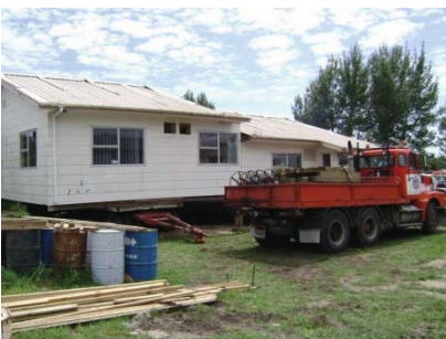
Piece 1 and 2 admin building
