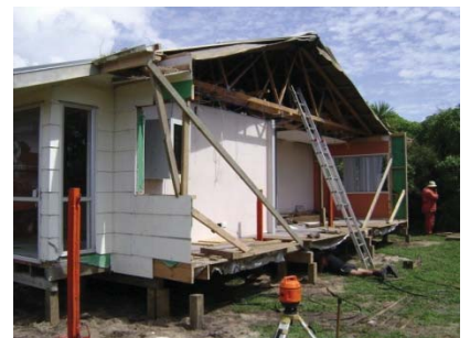
Part of the administration building
